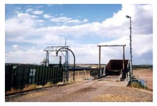
Truck-to-rail reload showing the truck dump, Fort Apache Timber Company, Snowflake, AZ. Source: USDA Forest Service
