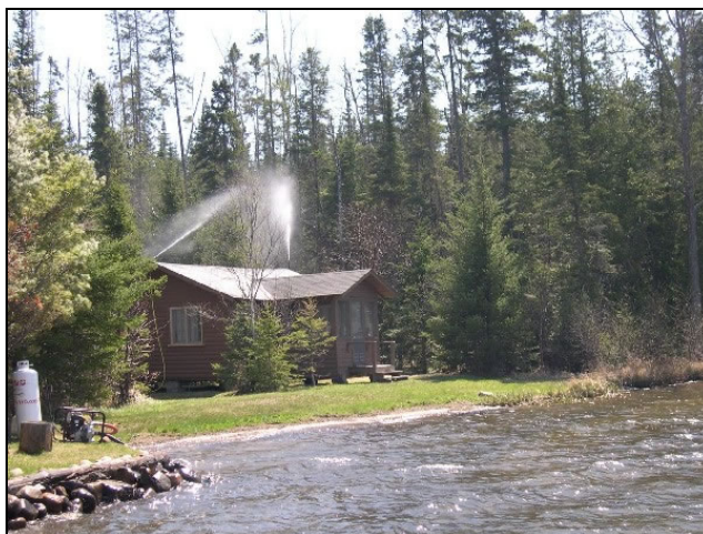
Image 3 Sprinkler system at private residence in Minnesota
