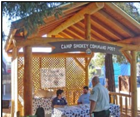
The Camp Smokey Command Post, built with small roundwood logs obtained from hazardous fuels projects in northern California. (9-30-CA-3.tif)
