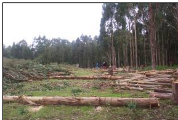
Hazardous fuel reduction is underway in the eucalyptus groves along Highway One near the communities of Olema and Bolinas, California.
