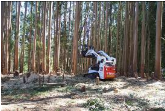
A bobcat is used to clear cut trees in the Highway One fuelbreak project.
