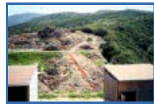
Completed section of fuel break with BLM border noted by dashed line.
