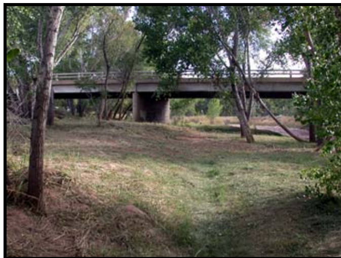
Looking at the finished product, an improved firebreak next to the bridge.
