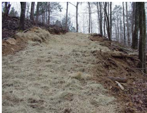
This fireline was mulched and seeded to minimize soil movement. Six weeks and six inches of rain (in a 24 hour period) later there was little soil movement.
