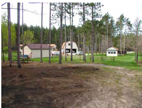
The wildfire never touched this home and outbuildings in Adams County, WI, because the homeowners created and maintained a defensible space. Photo courtesy WI DNR
