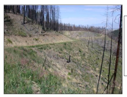
West Fork Wilson Creek prior to BAER work. Accelerated overland flow from the burned slopes above was eroding the cut slope and road surface and increasing sediment delivery potential to West Wilson Creek, a Westslope Cutthroat fishery.
