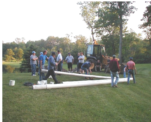
The Scotland Volunteer Fire Department installs a dry fire hydrant
