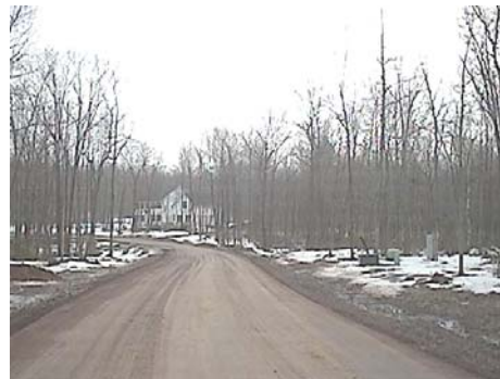
Laurelbrook: Road designed using Firewise Guidelines
