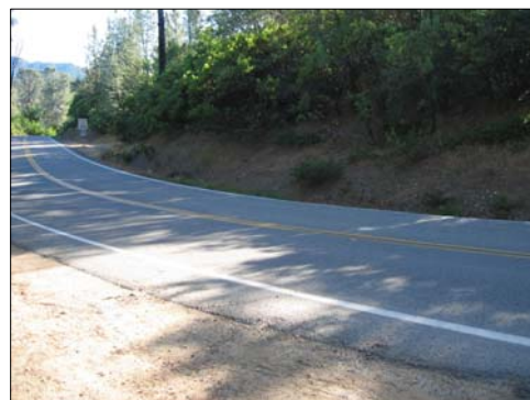
Rock Creek Road - Before
