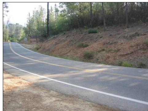
Rock Creek Road - After
