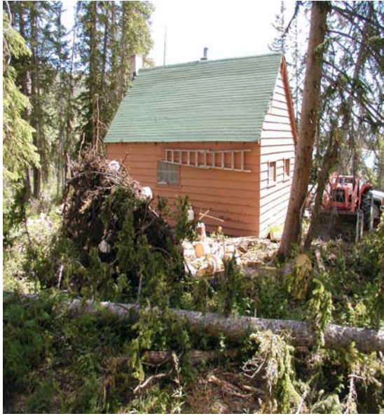
Private cabin where slash reduction work is in progress
