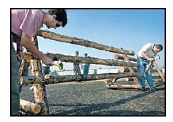
Patrick Ray, left, and Justin Maschhoff demonstrate the assembly of a buck and rail fence designed to make good use out of small-diameter logs thinned from forestlands.
