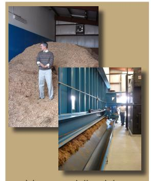
Wood chips are moved efficiently from a stockpile, via an automated conveyor sytem, to the biomass boiler where they become the source of fuel for the Ely School's heating system.
