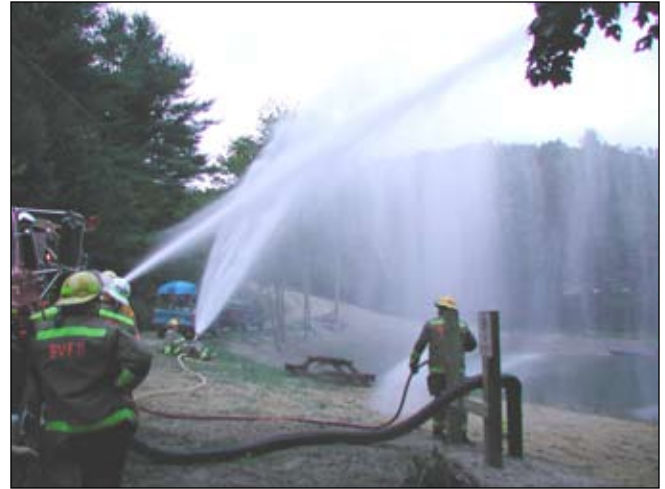
The Bridgewater VT Fire Department conducts a flow test on a dry hydrant installed in a pond.
